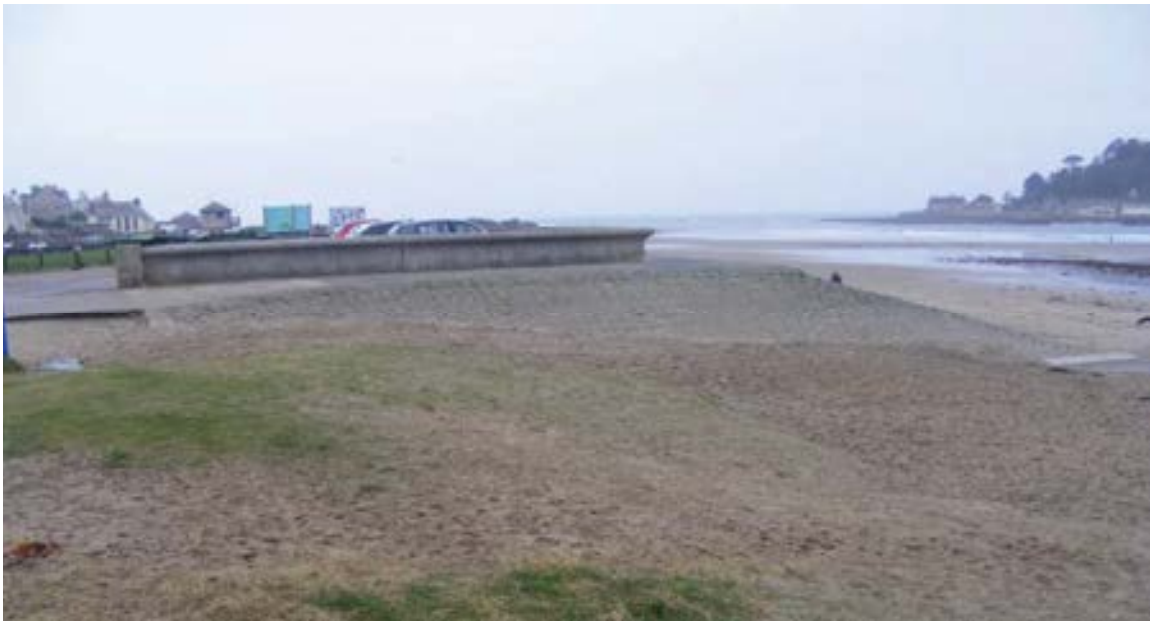
Figure A.6 Point where sand dunes to east of Red River (and in front of car park) meet seawall and rock armour frontage which protect Marazion town. This is a key access point from the car park to the dunes and beach (taken during site visit 1 st February, looking south east).
