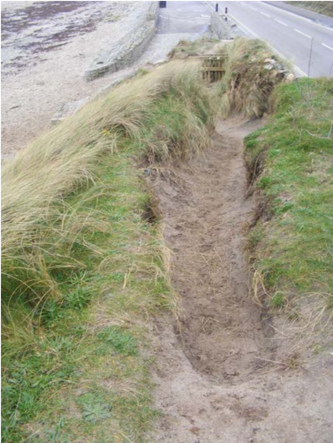
Figure 2.3 Footpath erosion at western end of dunes.
